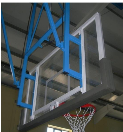
Fig. 2 Drop down goal support structure example
